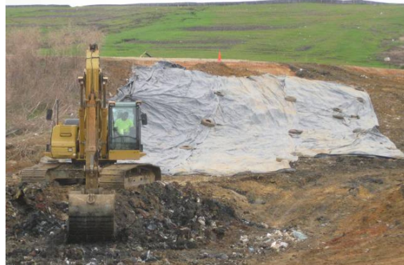
Figure 6. Covering the Exposed Waste Surfaces
