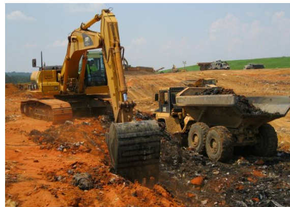
Figure 2. Waste Excavation and Transportation Operation
