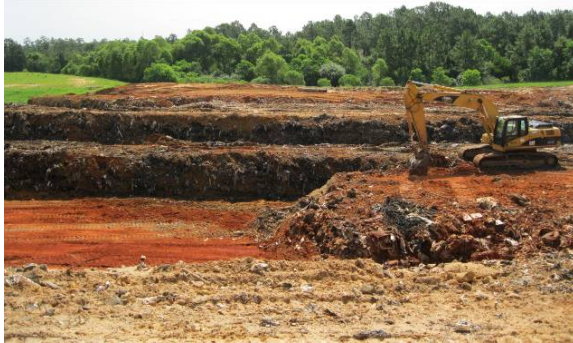
Figure 3. Steps Resulting from Waste Excavation
